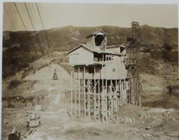
POW Camp 18B, Yunoki, Kyushu, Japan View of Soto Dam showing cement mixer in foreground
