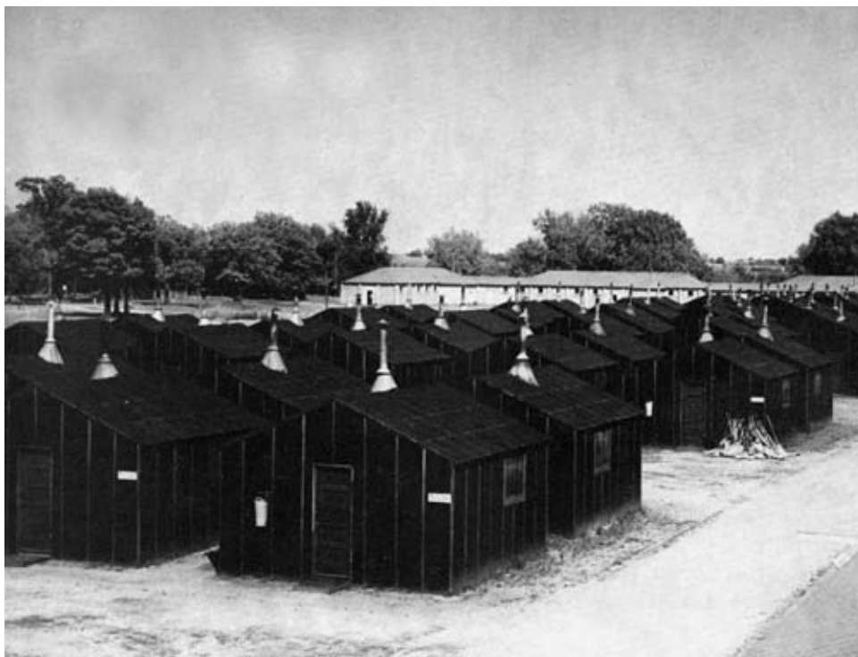
Temporary barracks known as the Turkey Farm
