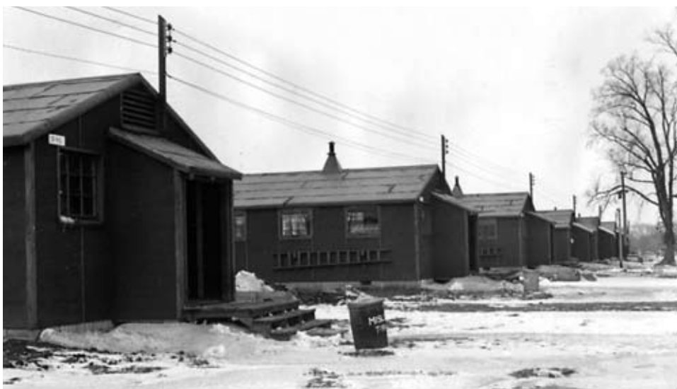
Temporary barracks at Camp Savage
